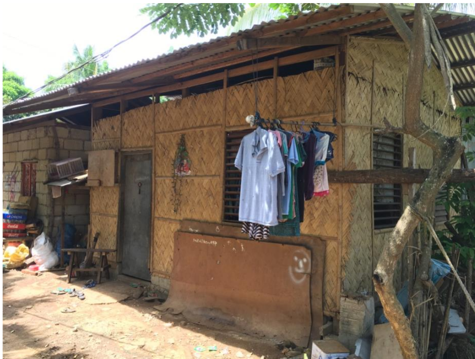
Figure 1. The house of one of my informants in New Princesa with concrete flooring and local coconut fibers used for the walls. Corrugated steel is commonly used for roofing.
